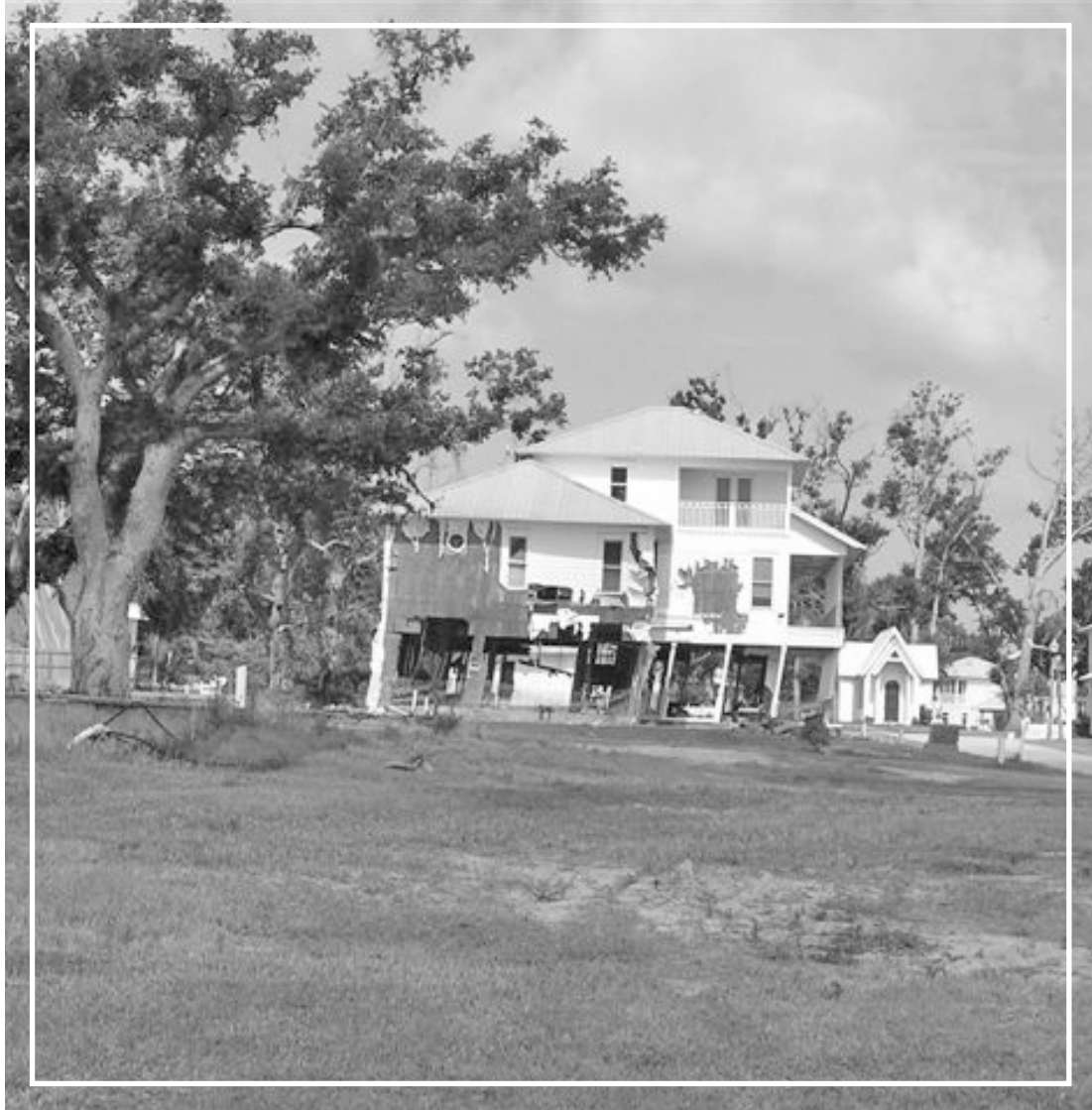
A stately Louisiana Gulf Coast home awaits repairs.
