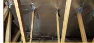
**Radiant Barrier Insulation**
