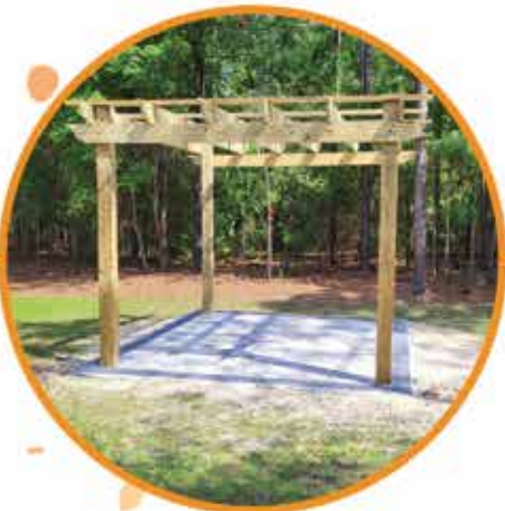
Pergolas, Pavers & Stack Walls
